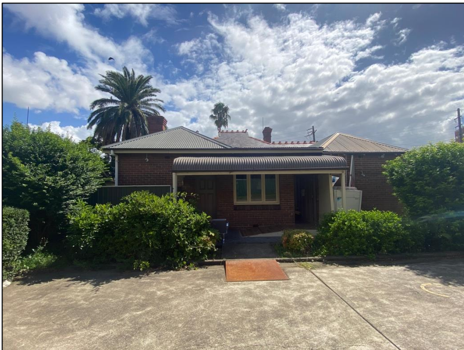
Figure 18: No. 62 Railway Parade. Rear wing showing hipped roof to either side of the skillion.
